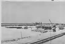
Dredging and land reclamation work started April 2, 1969.
